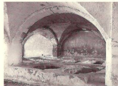
5. Interior of «Cal Granotes» before its rehabilitation.
